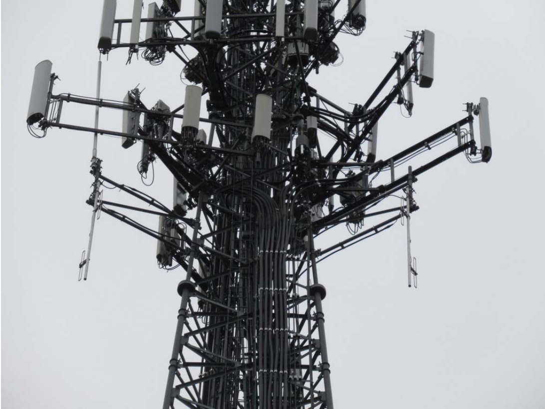
Photo 1: Photo illustrating the Tower with Appurtenances shown.
