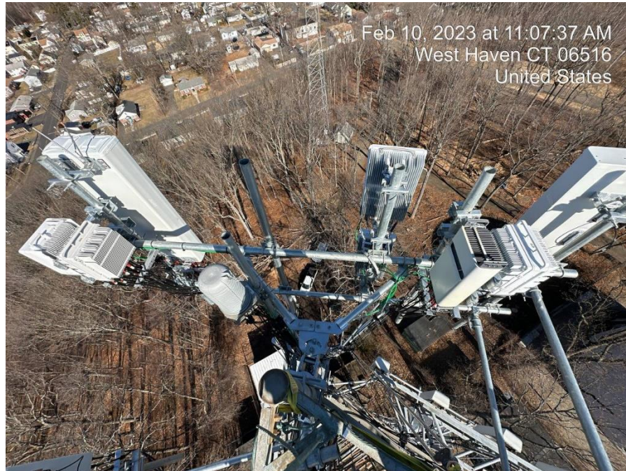
Photo - 1: Installation of proposed antennas & equipment
