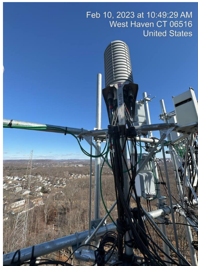
Photo - 2: Installation of proposed antenna mount
