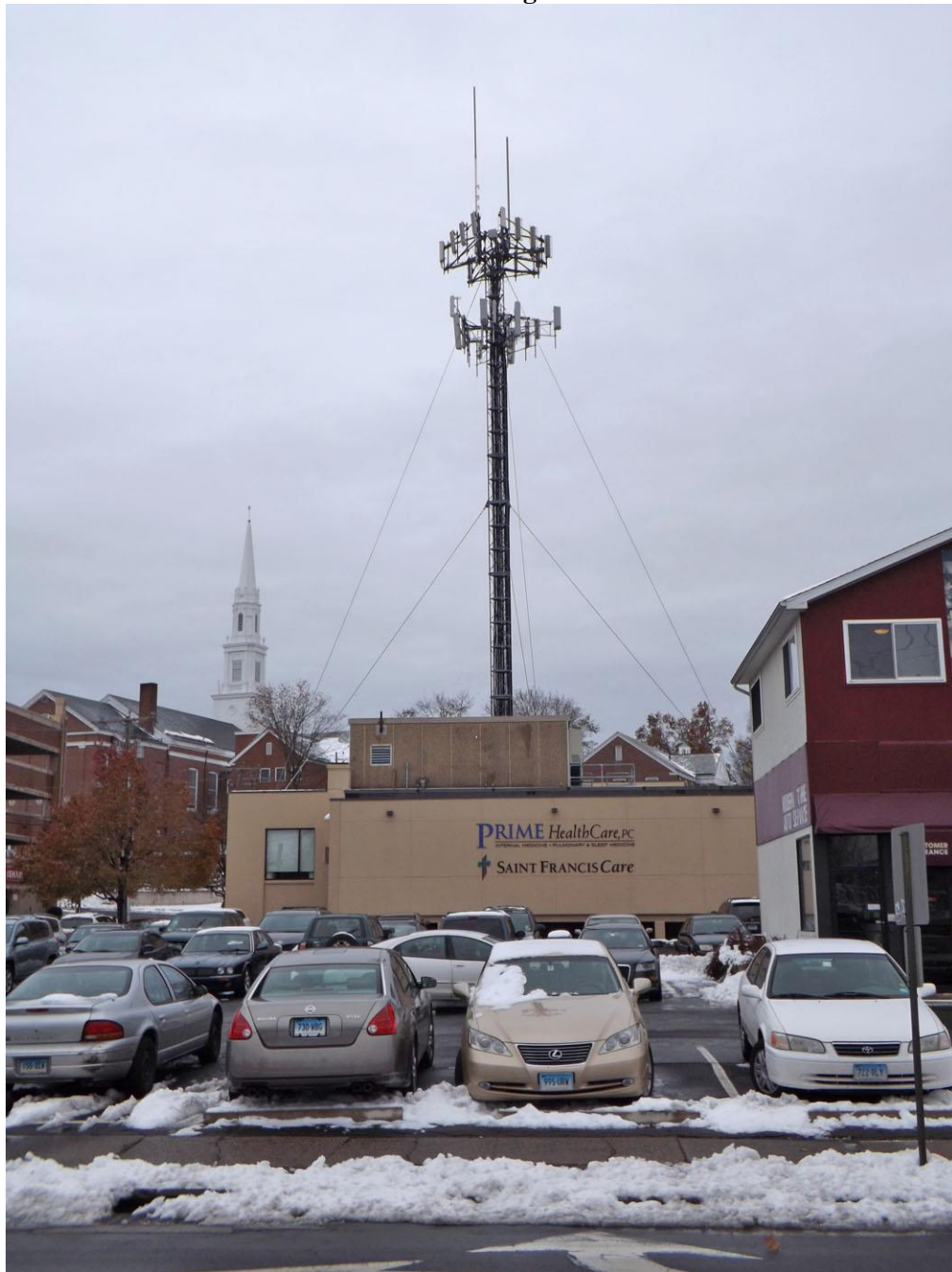
View of Existing Tower
