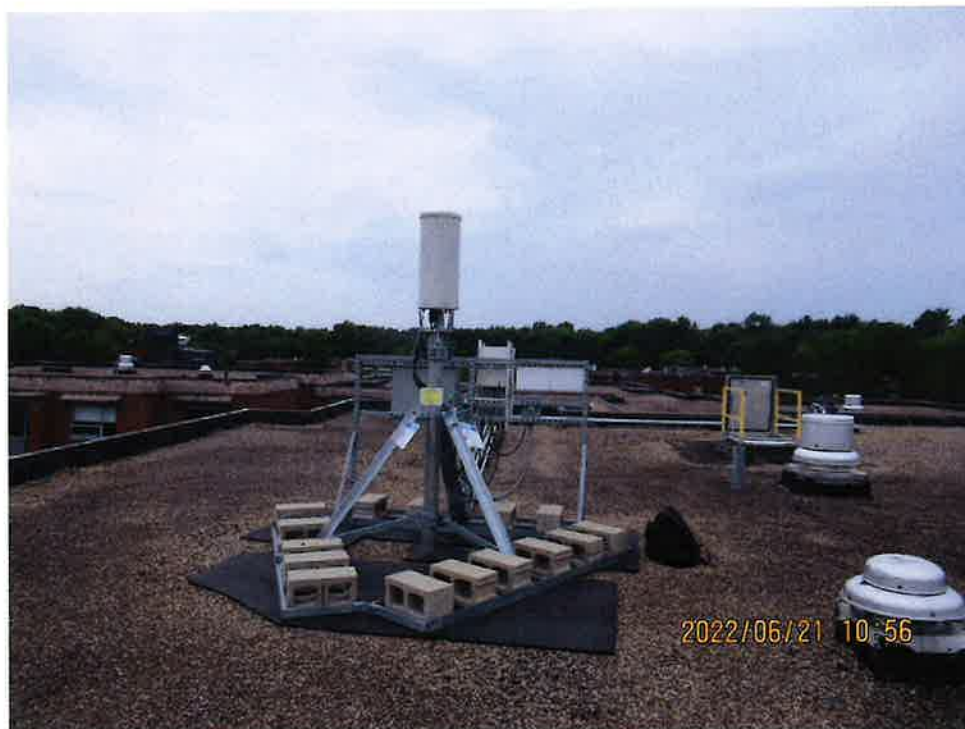
Photo 2: Sample photo illustrating the existing antenna and RRH.
