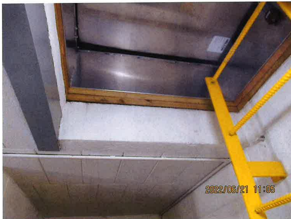
Photo 4: Sample photo illustrating the existing roof construction.
