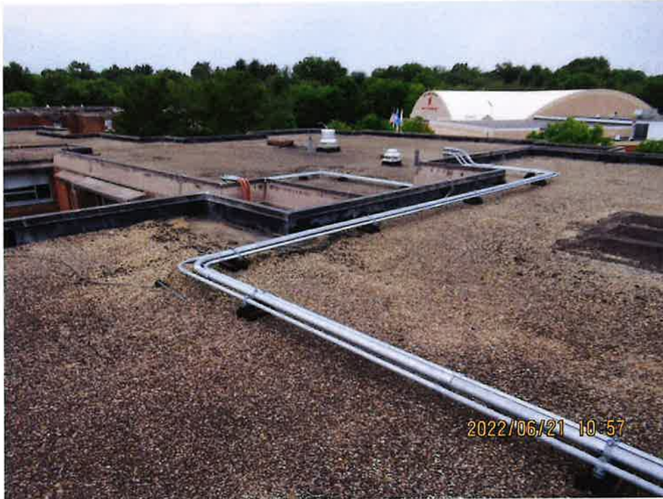
Photo 3: Sample photo illustrating the existing roof construction.
