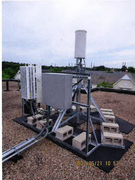
Photo 1: Sample photo illustrating the existing antenna and RRH.
