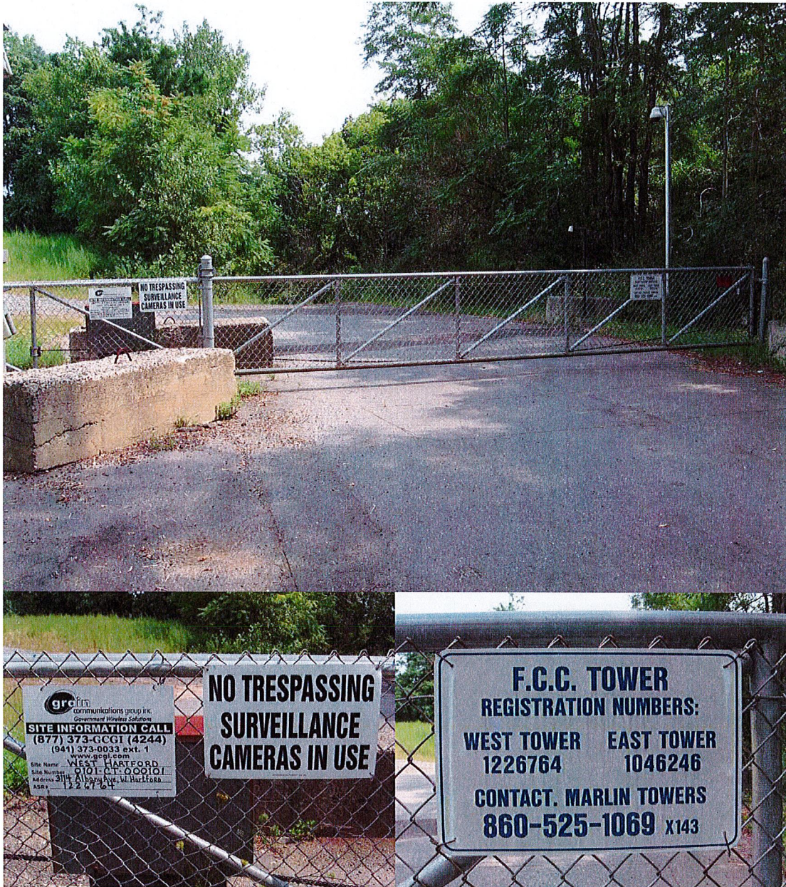
Figure 2: Tower Access Road Gate and Signage
