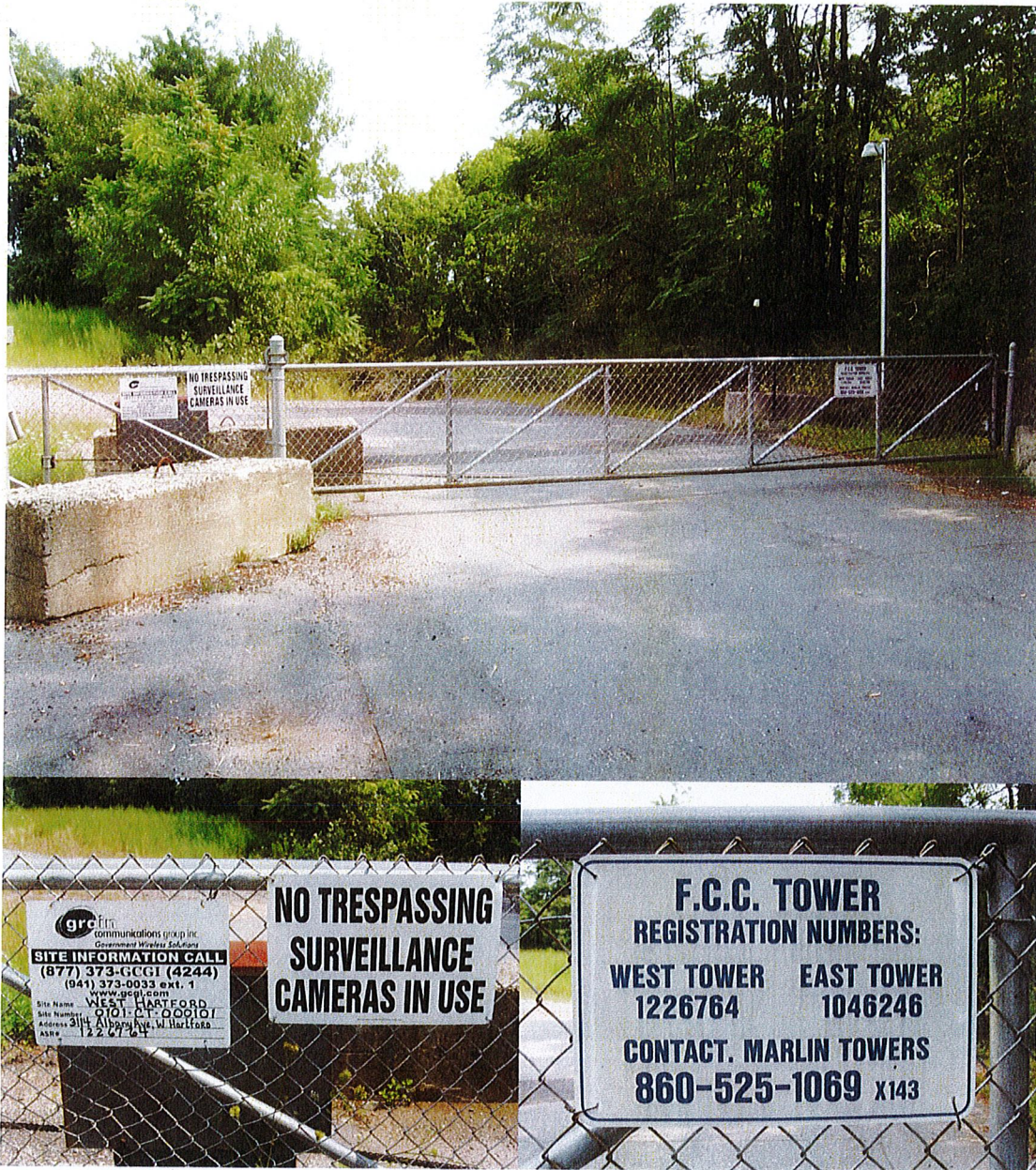
Figure 2: Tower Access Road Gate and Signage
