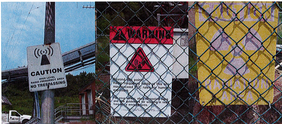
Figure 4: Compound Facility and RF Signage
