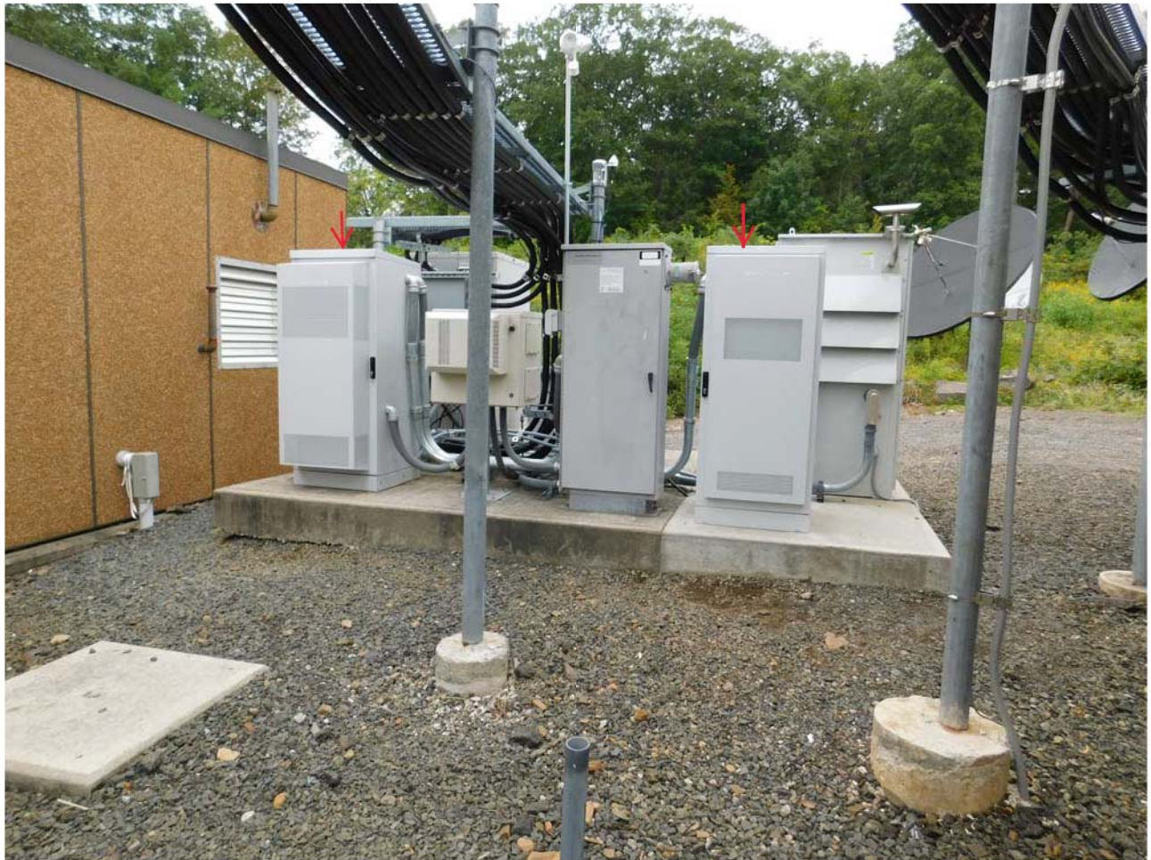
(2) New Equipment Cabinets Mounted To Existing Concrete Pad
