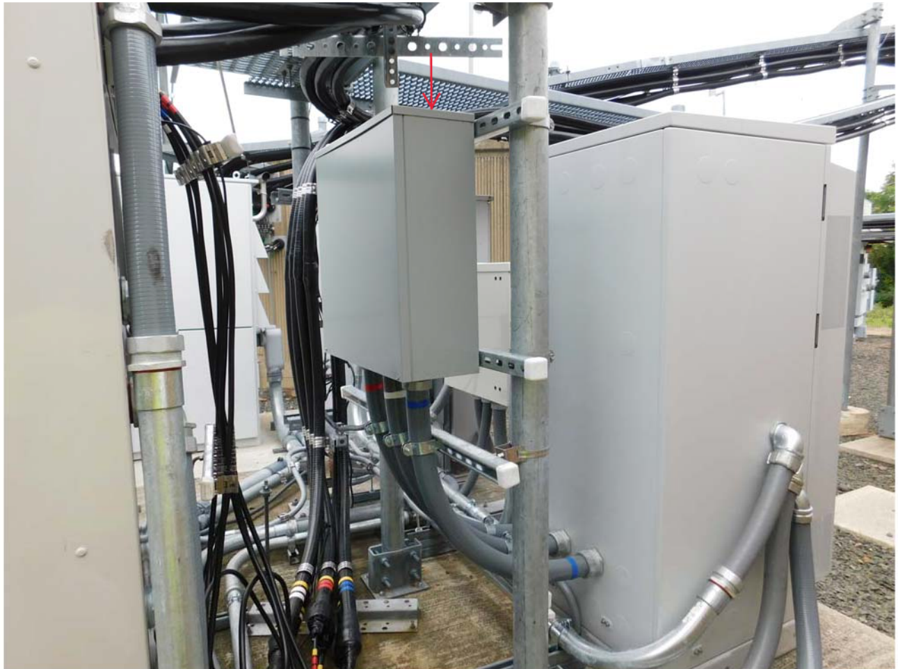
New Slack Box Mounted To Existing Ice Bridge Post
