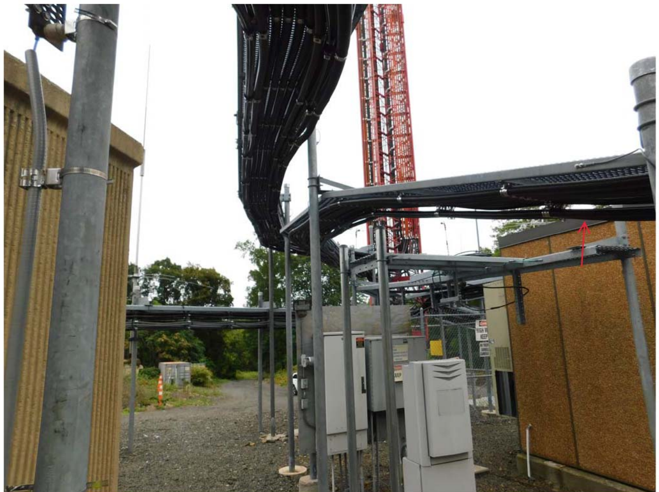
New Signal Cables Run Along Existing Cable Path
