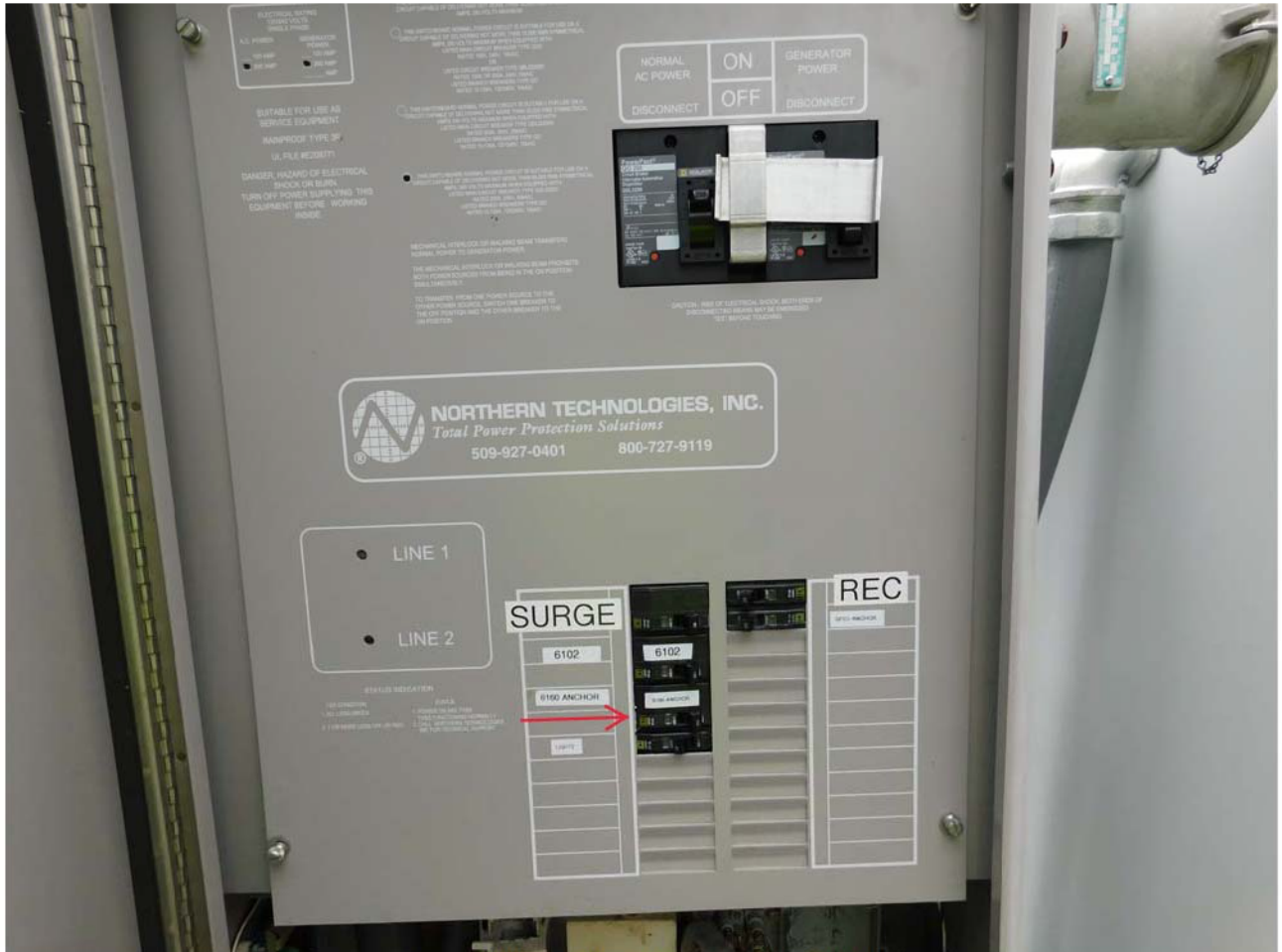
New Cabinets Tied Into Existing PPC
