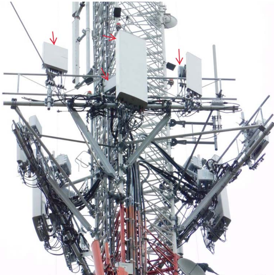
Beta Sector: (2) New Antennas, (3) New RRHs & Ancillary Equipment Mounted To Modified Sector Frame
