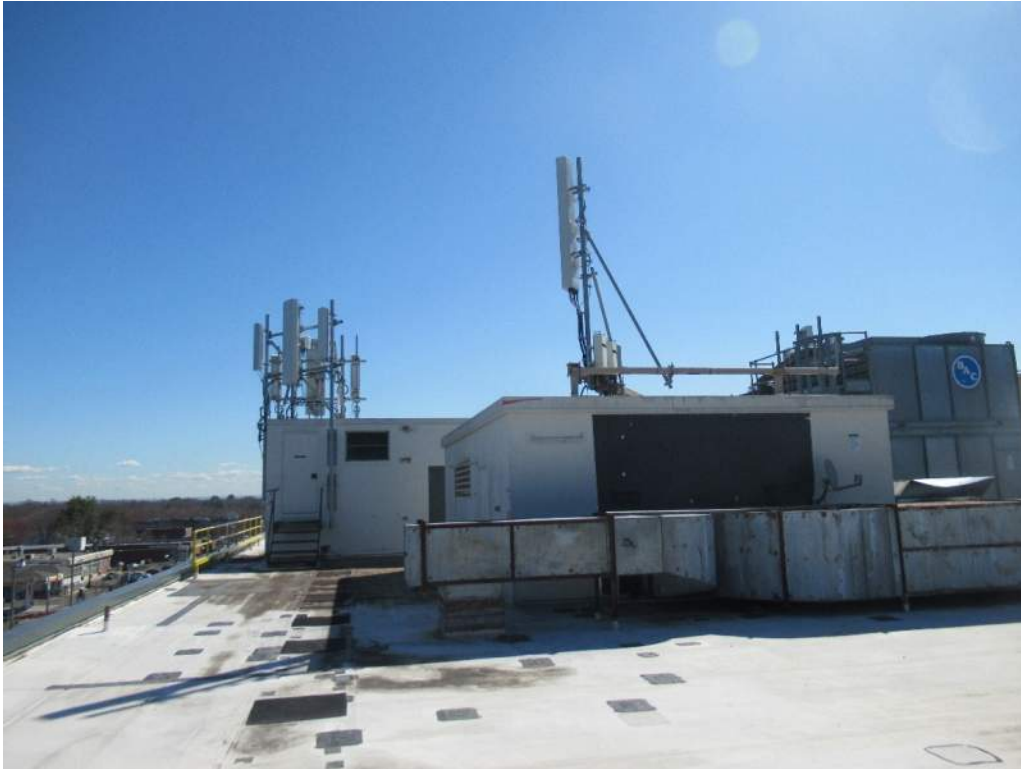
Photo 1: Sample photo illustrating the existing Alpha sector.
