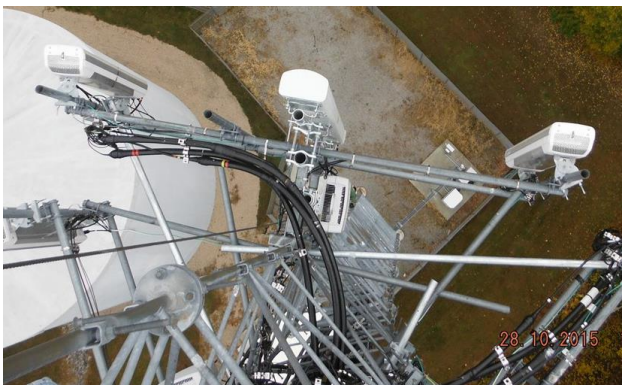
Typical sector from above (photo provided by contractor)
