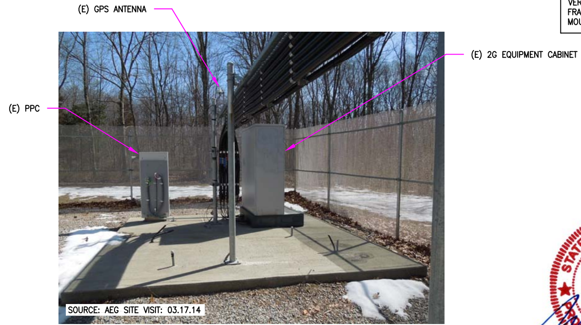
EXISTING EQUIPMENT AREA. N.T.S.
