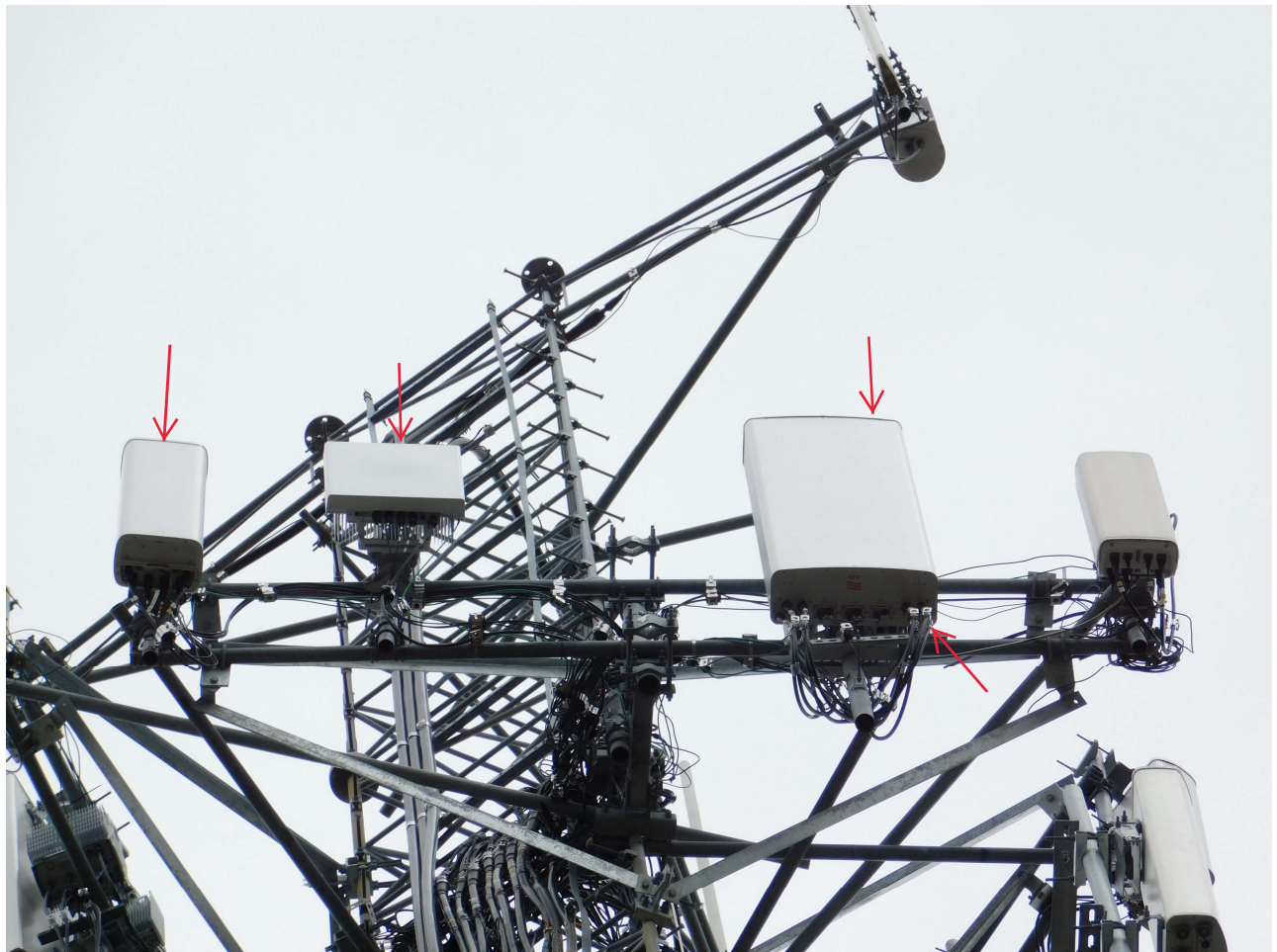
Beta Sector: (3) New Antennas & (2) New RRHs Mounted To Modified Sector Frame
