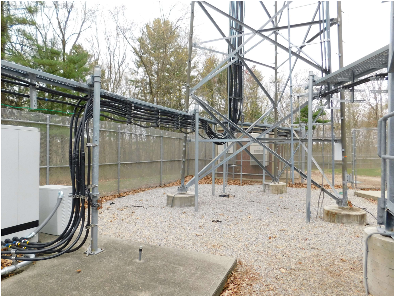
(9) New Signal Cables Routed Along The Existing Cable Path
