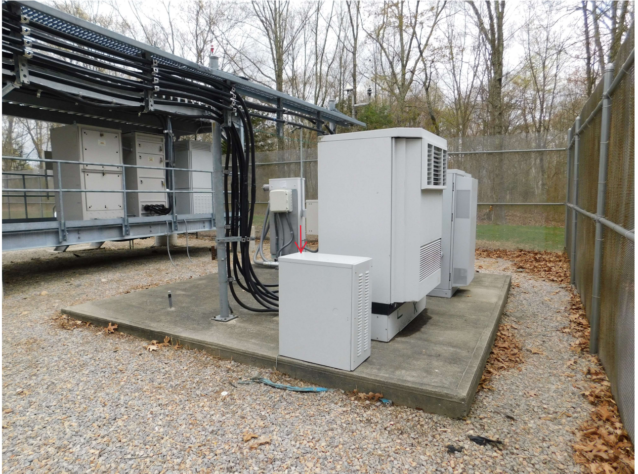
(1) New Cabinet Mounted to Existing Concrete Pad
