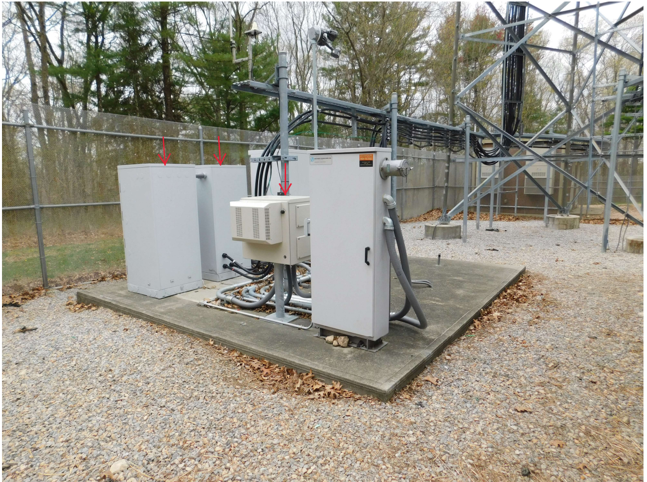
(3) New Cabinets Mounted to Existing Concrete Pad
