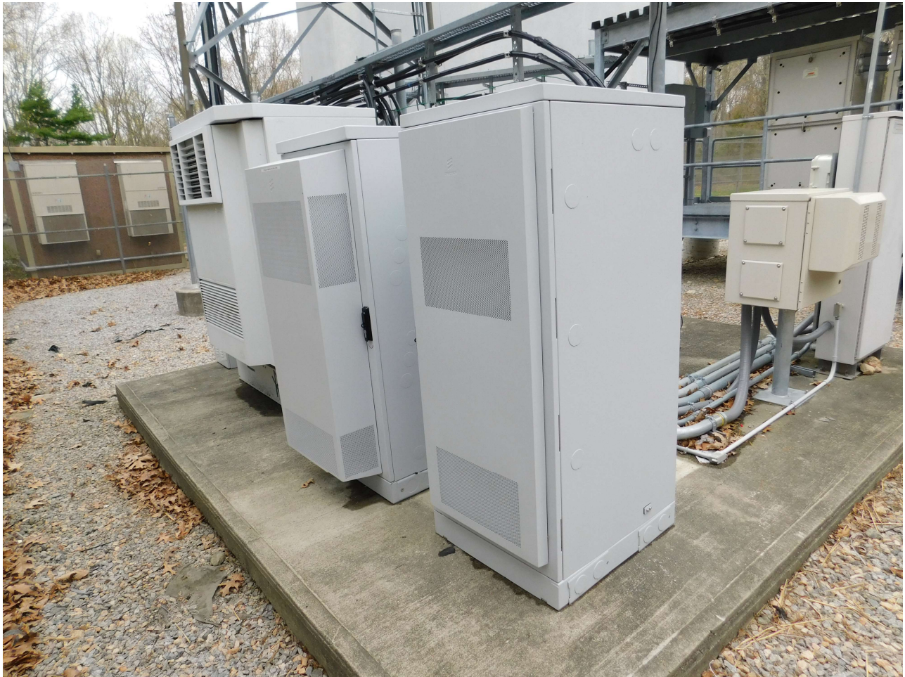
New Equipment Cabinet & Battery Cabinet Mounted to Existing Concrete Pad
