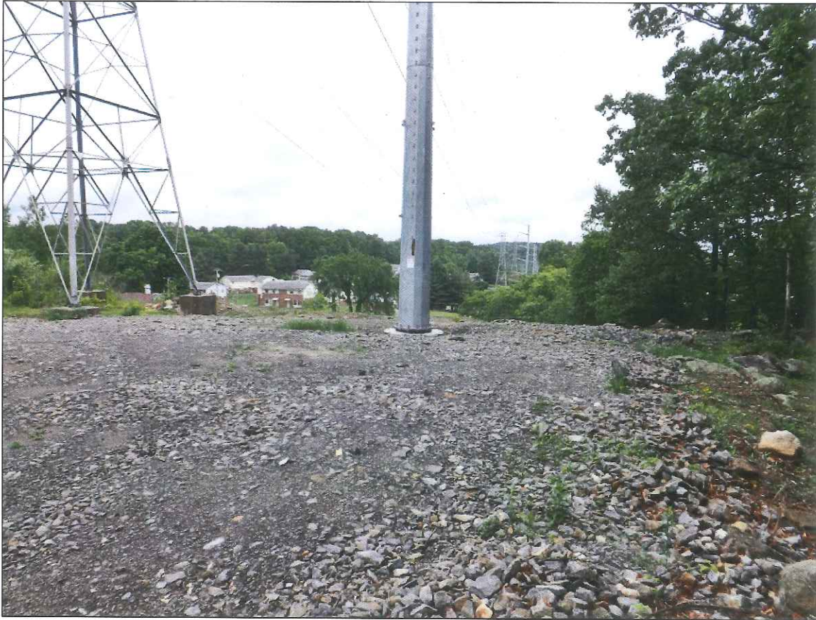
Site of equipment compound
