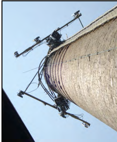
Existing antenna mounts & smokestack
