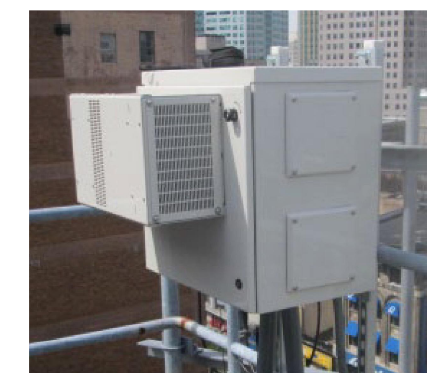
EMERSON NETXTEND COMPACT 2416 AAV CABINET DIMENSIONS: 24.0"H x 25.25"W x 25.24"D TOTAL OF 1
