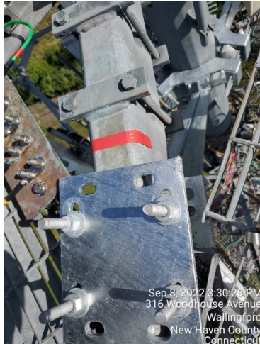
Top Brace Connection to Ex. Mount
