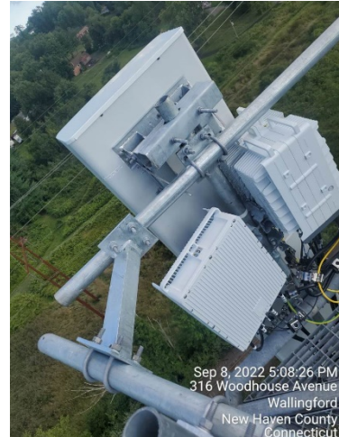
AHCP Corner Plate Kit Installed
