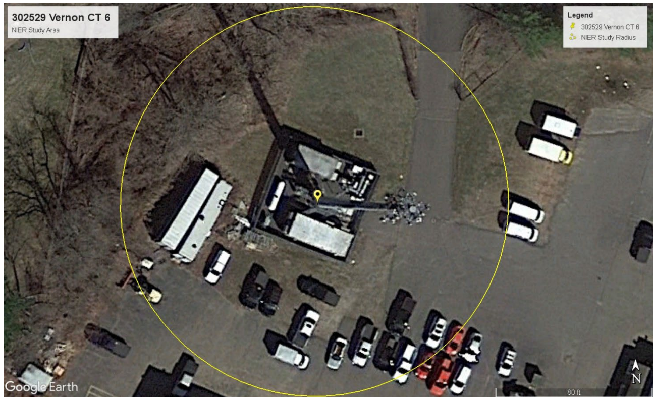
Aerial View of Site
