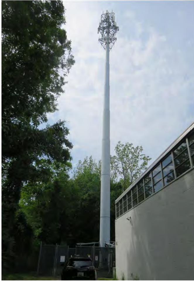
FULL VIEW OF TOWER
