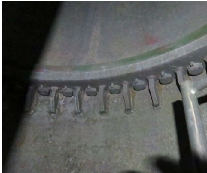
INSIDE TOWER JOINT 3
