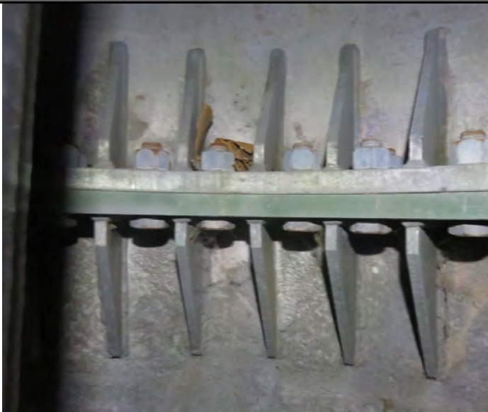
INSIDE TOWER JOINT 2
