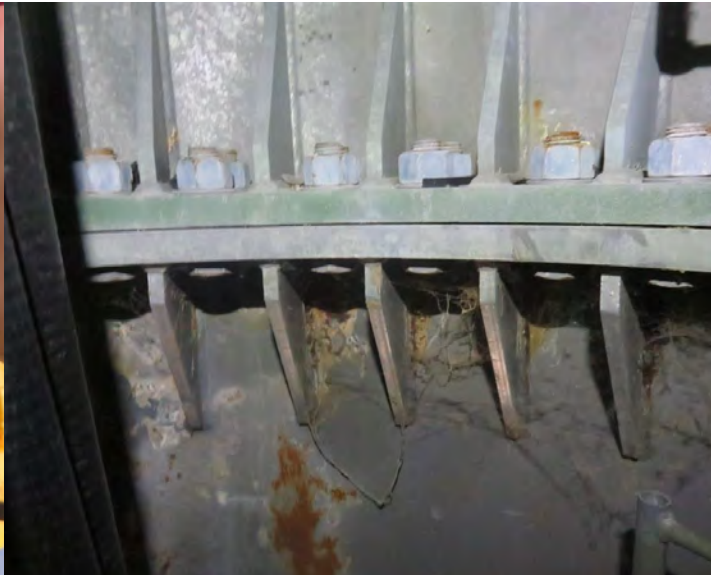
INSIDE TOWER JOINT 1
