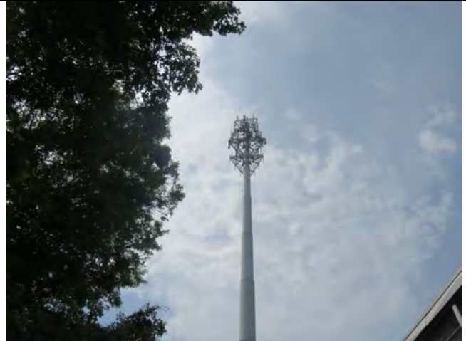
TOP HALF OF TOWER
