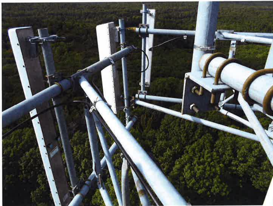
Photos of Verizon's existing panel antennas.
