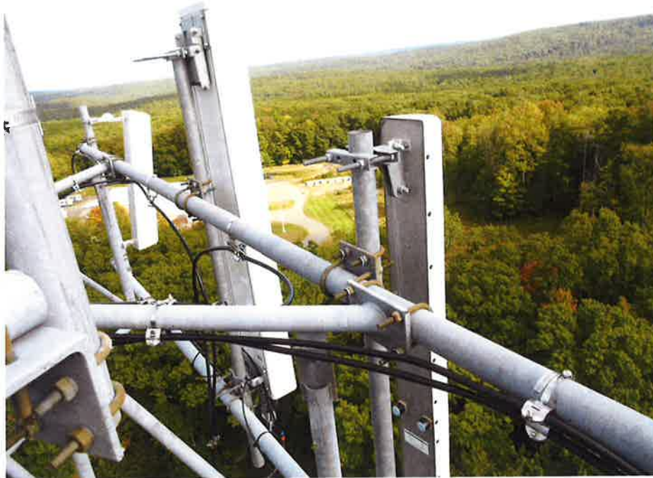
Photo of Verizon's existing panel antennas.
