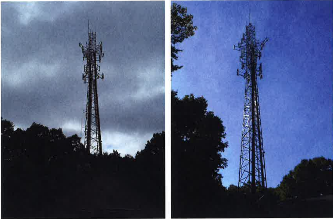
Overview photos of 180' self-supporting tower.
