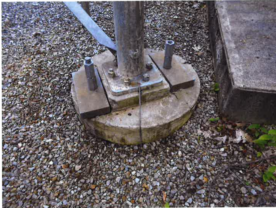
Photo of typical foundation pier.
