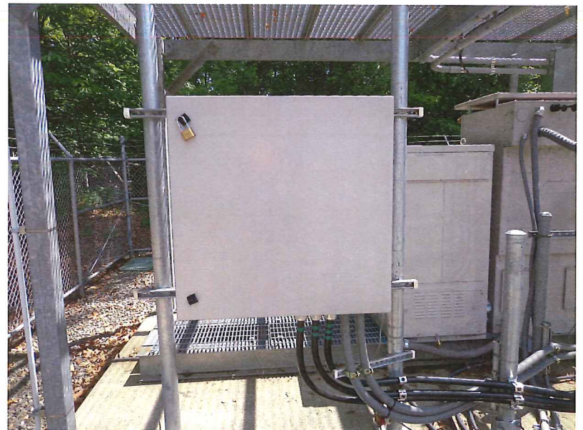
4 EXIST FIBER DISTRIBUTION BOX SCALE: NTS
