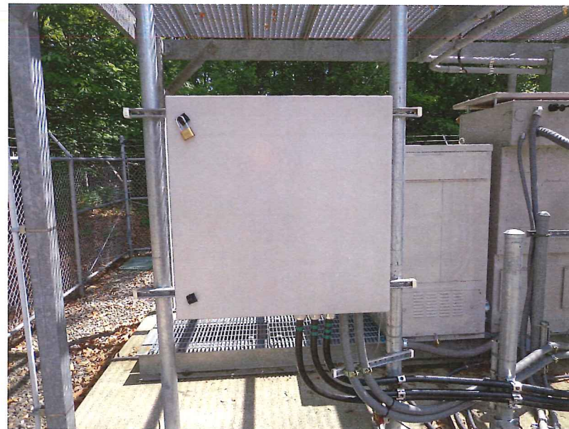
4 EXIST FIBER DISTRIBUTION BOX SCALE: NTS
