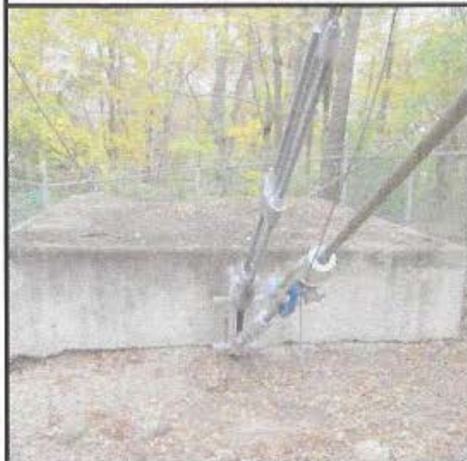
GUY ANCHOR CONFIGURATION (B & C PATH)
