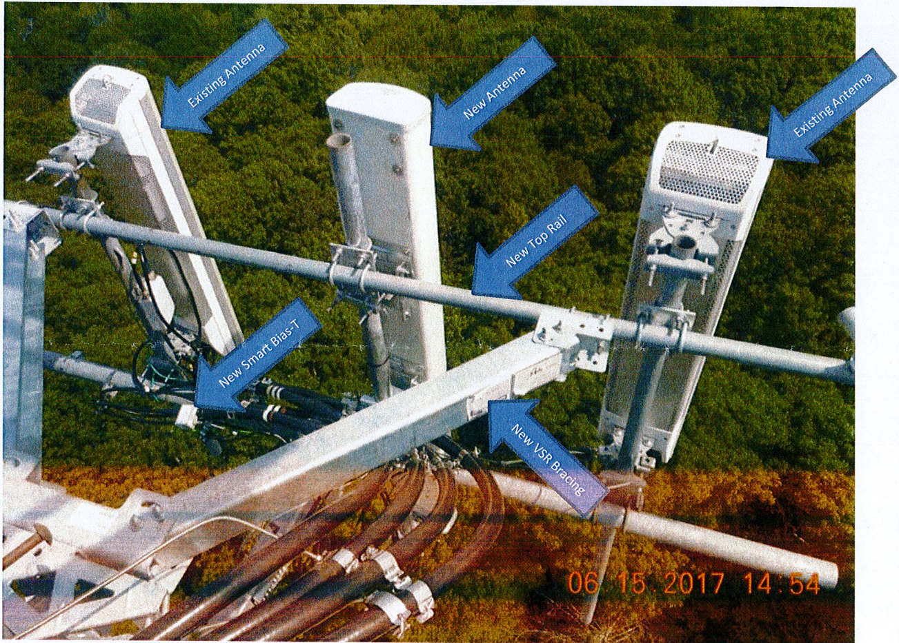
Typical antenna array with new antenna & sector reinforcement installed.
