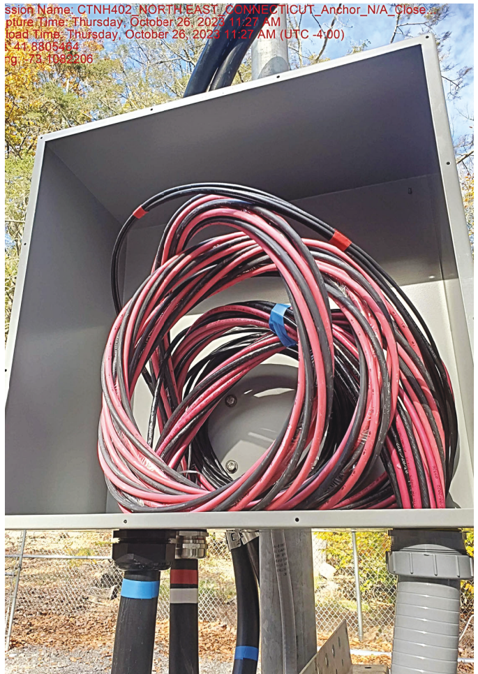
Slack box installed on ice bridge post
