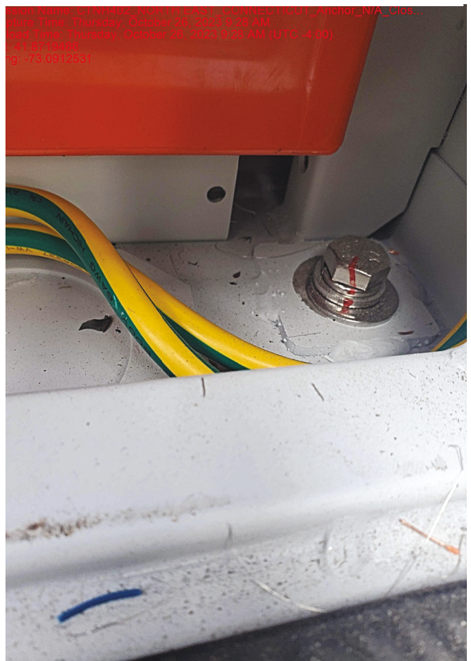
Typical anchoring of cabinet to concrete pad
