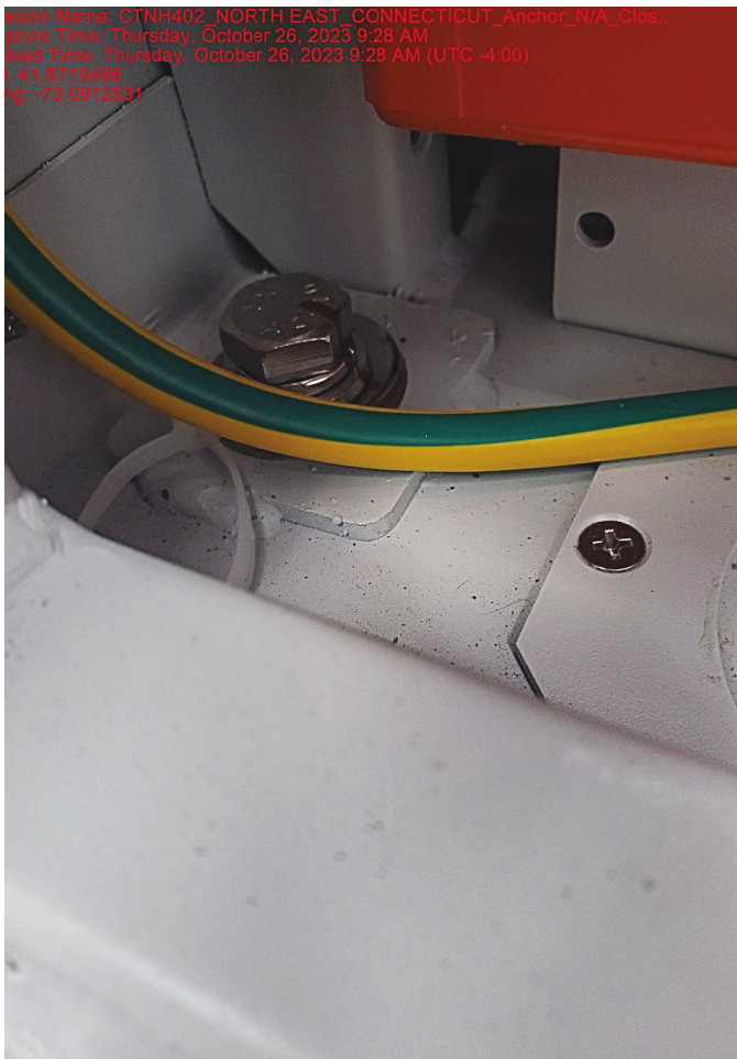
Typical anchoring of cabinet to concrete pad
