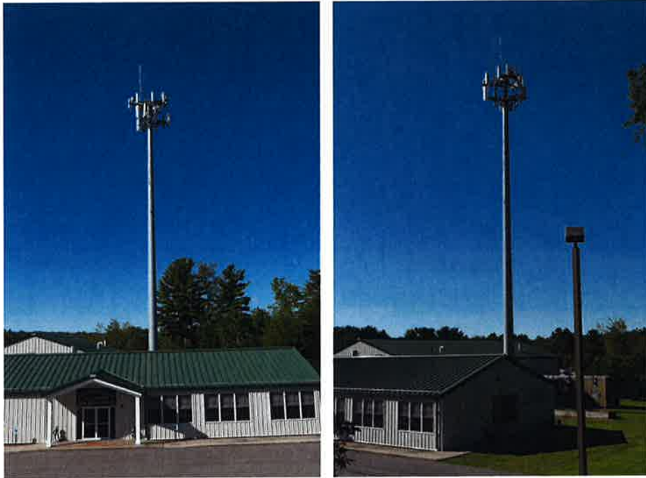
Overview photos of 125' monopole tower.
