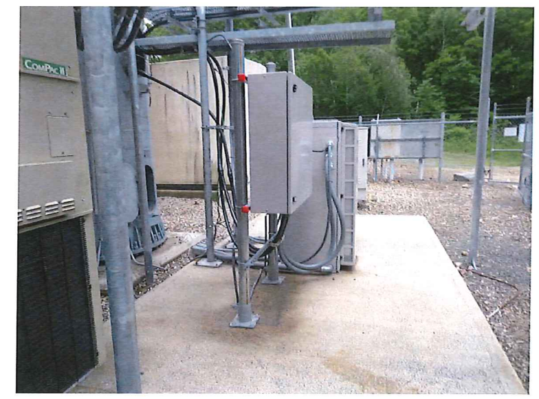
4 EXIST FIBER DISTRIBUTION BOX A-3 SCALE: NTS
