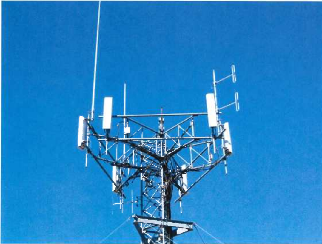
Photo 1: Photo illustrating the Tower with Appurtenances shown.
