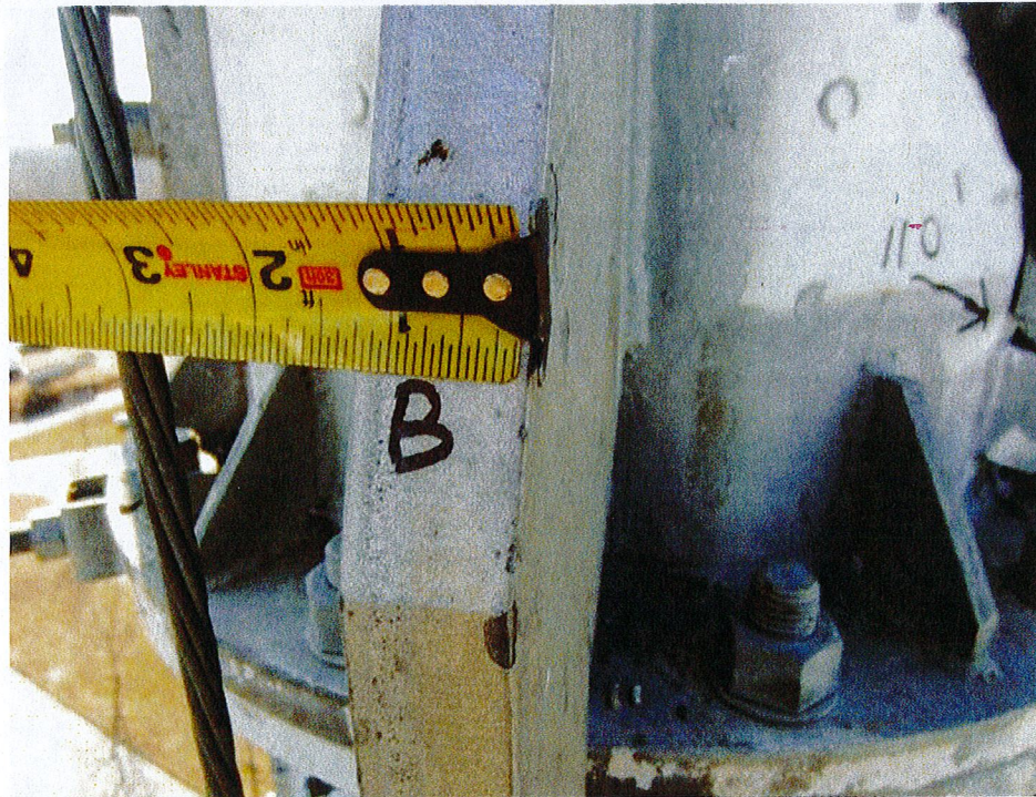
Verification of new 1-1/4" thick bridge stiffener
