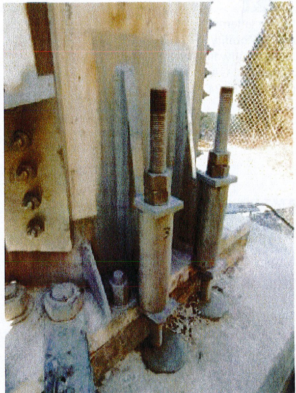
New 1-1/2"Ø fully threaded anchor rod (Typ 8)
