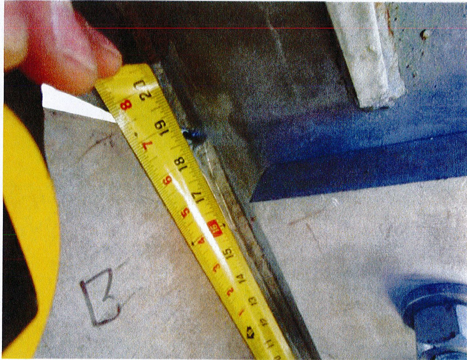
Verification of 18" connection point to tower
