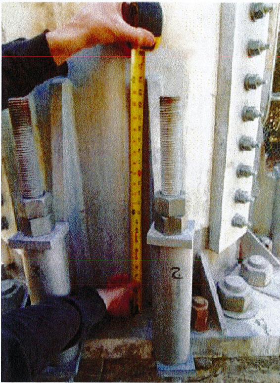
Verification of 24" tall anchor rod bracket
