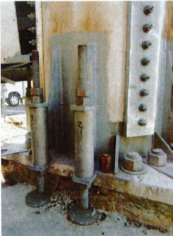
New 1-1/2"Ø fully threaded anchor rod (Typ 8)
