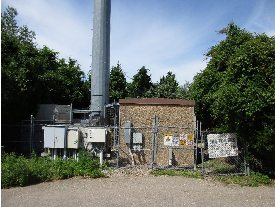
Figure 1: View of ES-026 Stonington
