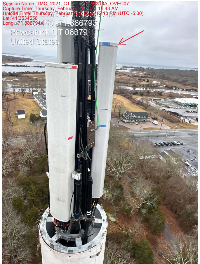
Gamma Sector: (1) New Antenna Mounted To Existing Unipole
