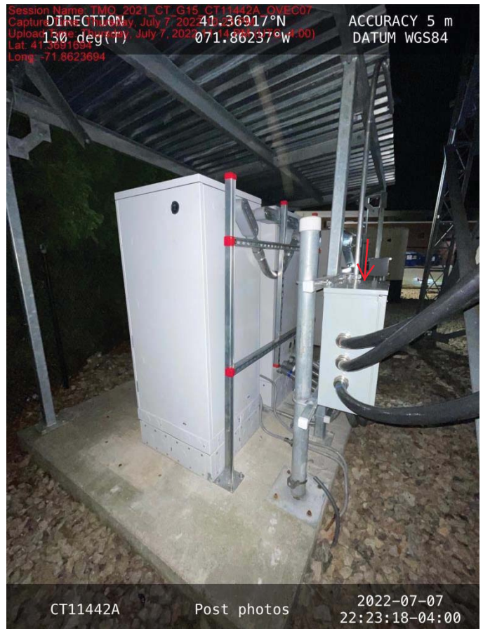
New Slack Box Mounted To New H-Frame
