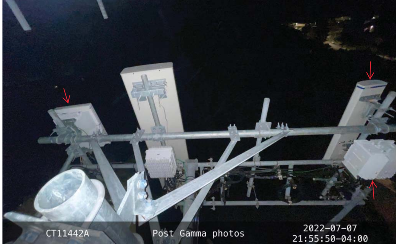
Gamma Sector: (2) New Antennas & (1) New RRH Mounted To Modified Sector Frame
