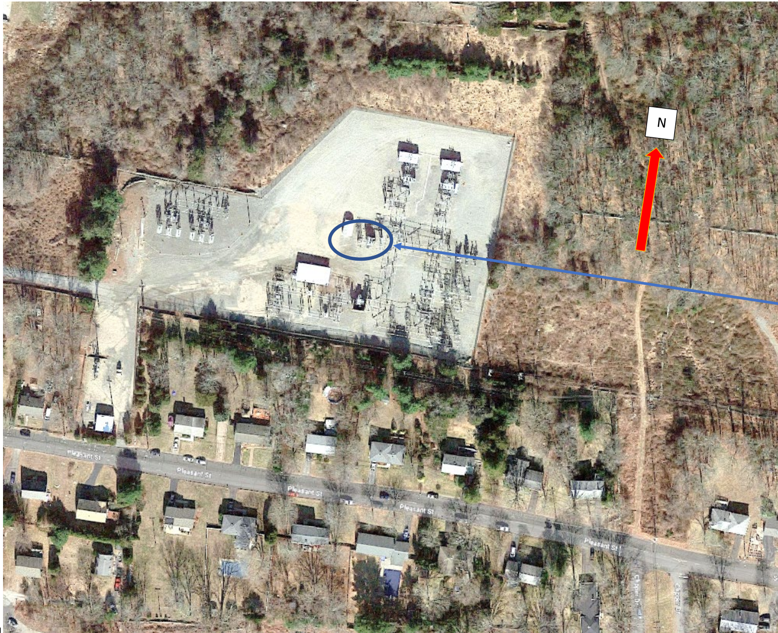
Mystic Substation, 148 Greenmanville Ave, Mystic, CT
