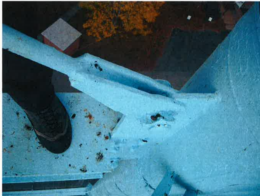
Photos of existing bracing connection.
