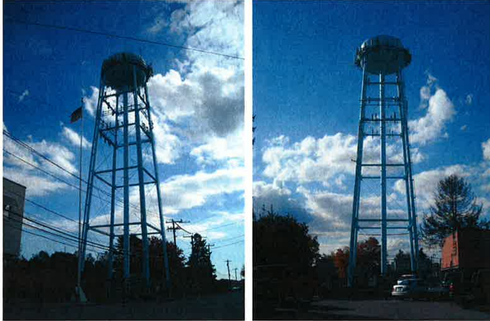
Overview photos of 155' water tank.
