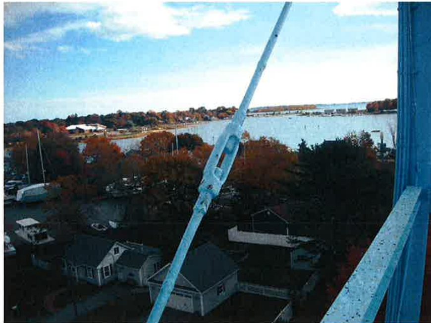
Photo of turnbuckle on existing brace.
