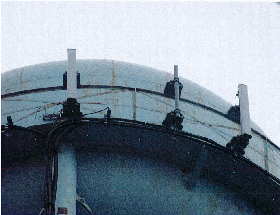
Figure 4: AT&T Mobility, LLC Proposed Microwave Antenna #41 (to right)
