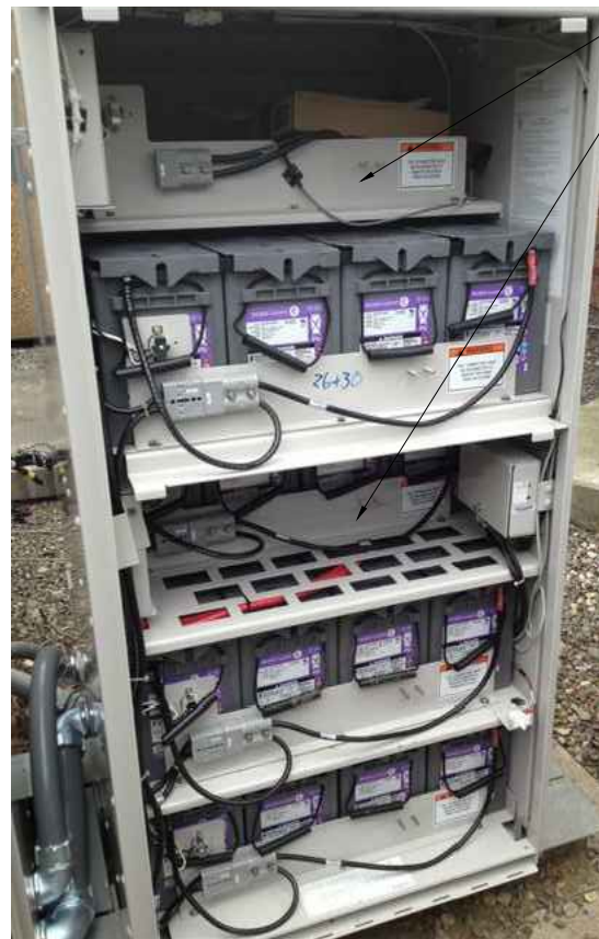
EXISTING BBU CABINET SCALE: NTS
