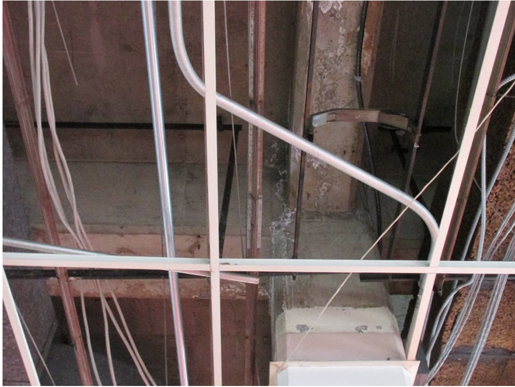
Building Construction (Interior Column)
