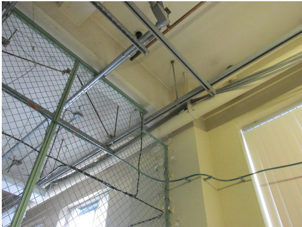
Building Construction (Exterior Column)
