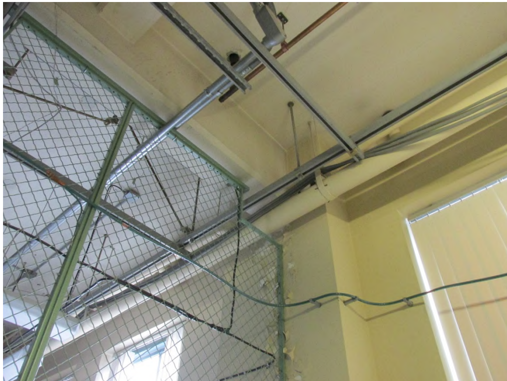
Building Construction (Exterior Column)
