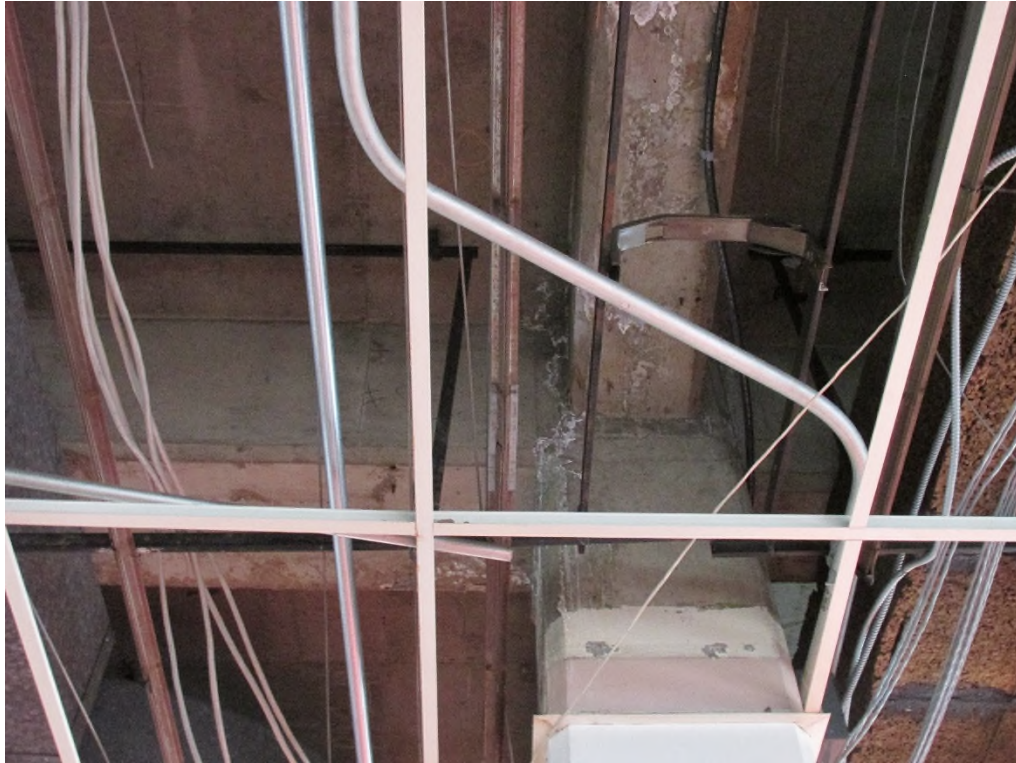
Building Construction (Interior Column)
