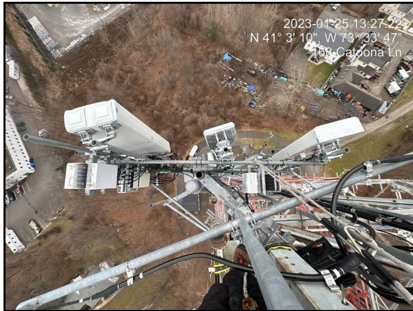
Figure 2: View of installed beta sector antennas and RRUs on existing sector frame
