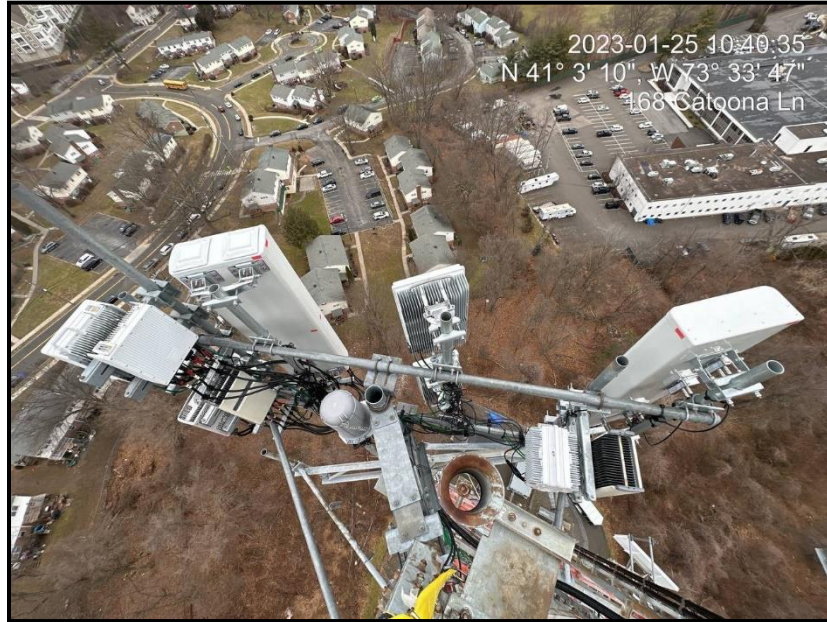
Figure 1: View of installed alpha sector antennas and RRUs on existing sector frame
