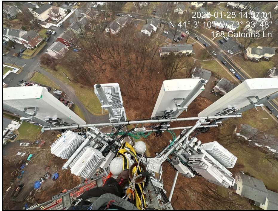
Figure 3: View of installed gamma sector antennas and RRUs on existing sector frame
