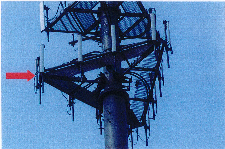
AT&T ARRAY TO BE REMOVED, SHOWN AT BOTTOM AT 123 FOOT LEVEL
