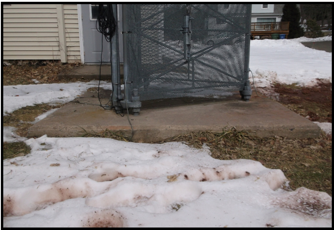
4) VIEW OF FOUNDATION AT GROUND SURFACE
