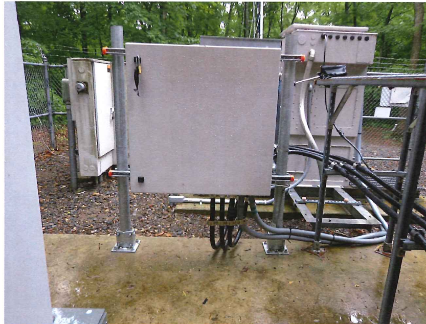
4 EXIST FIBER DISTRIBUTION BOX SCALE: NTS
