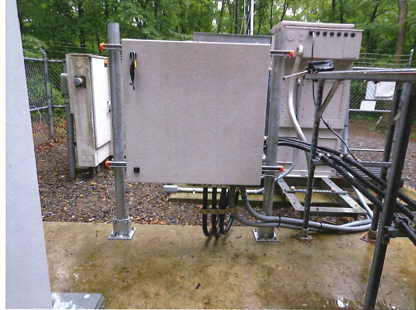
4 EXIST FIBER DISTRIBUTION BOX SCALE: NTS
