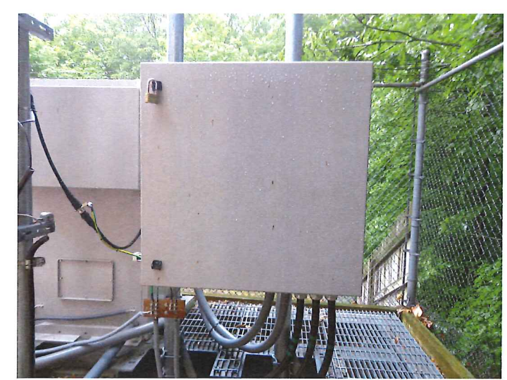
4 EXIST FIBER DISTRIBUTION BOX A-3 SCALE: NTS
