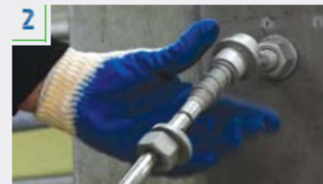
Remove the nut, the face washer and the spring shear sleeve and slide along the handle of the tool.
