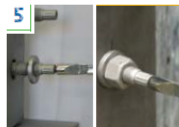
Slide the face washer forward and move the nut up to fasten to the bolt. Tighten the nut snug tight at this point.
