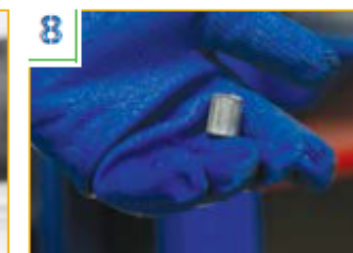
Press the small trigger on the shear wrench to eject the bolt spline. The application is now complete.
