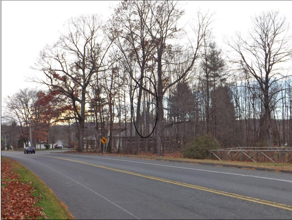
View of tower from north along Bushy Hill Road
