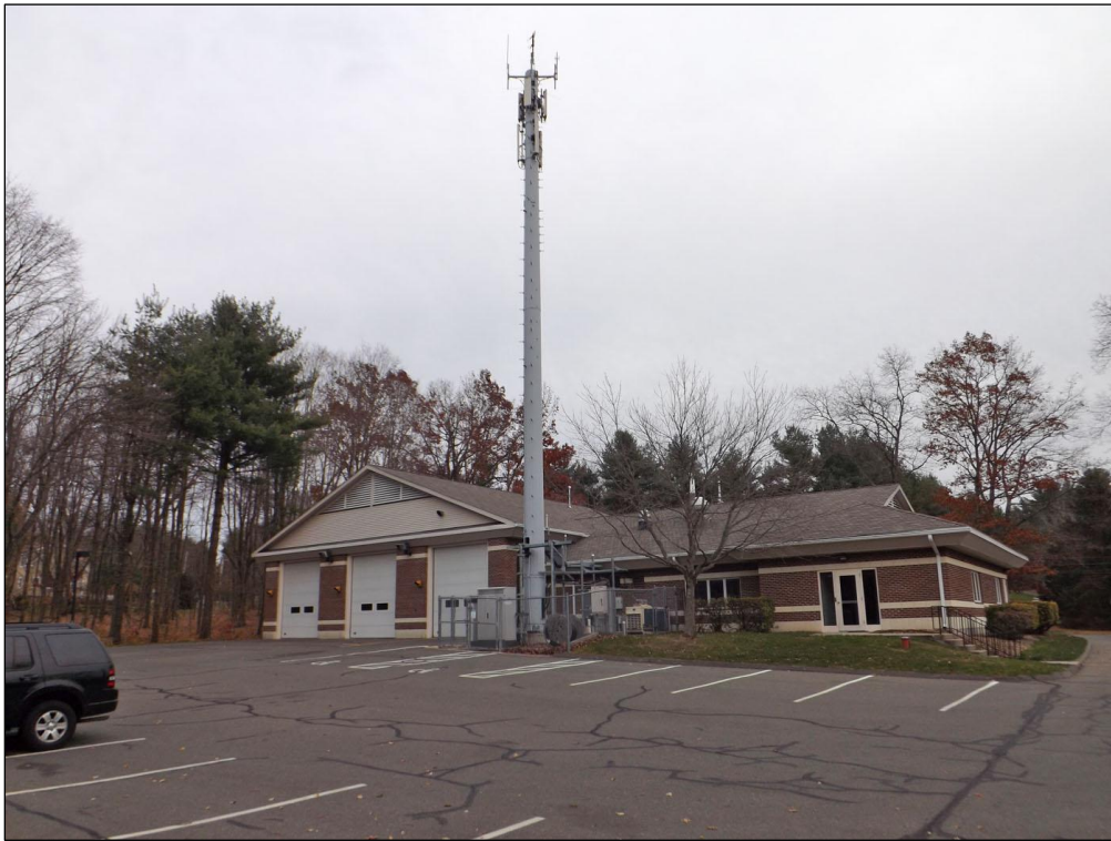
View of existing tower from behind fire house
