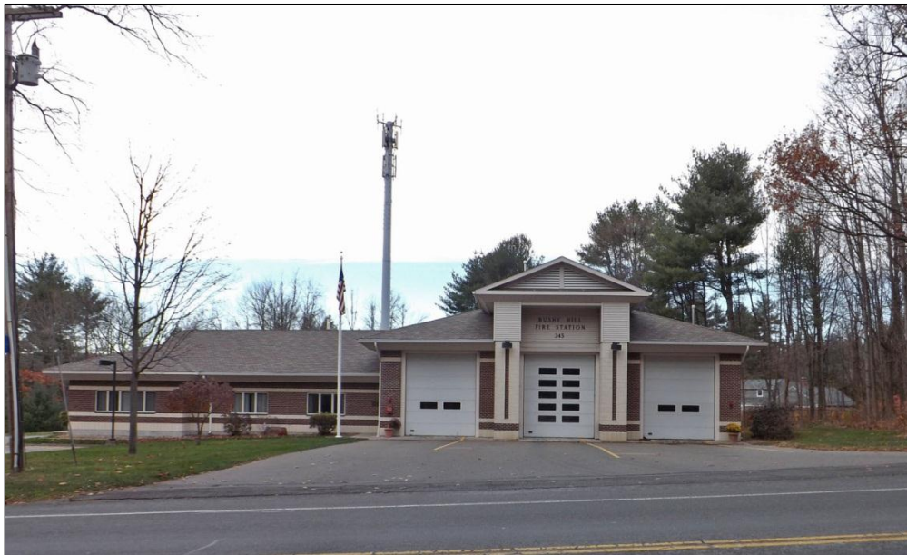
View of existing tower from across Bushy Hill Road
