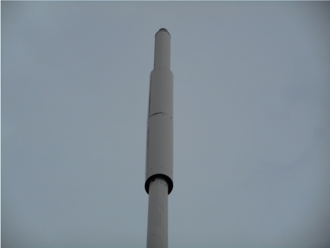
Photo 1: Photo illustrating the Flagpole with Appurtenances shown.
