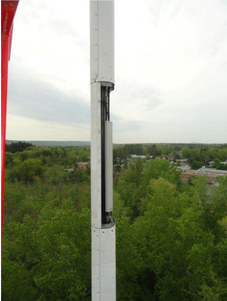
Photo 1: Photo illustrating the Flagpole with Appurtenances shown.
