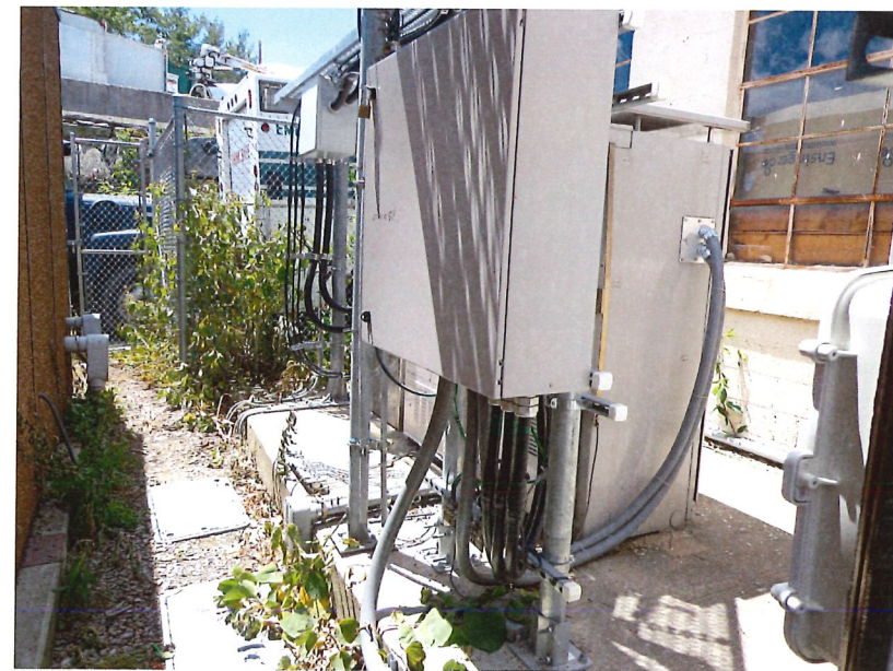
4 EXIST FIBER DISTRIBUTION BOX SCALE: NTS
