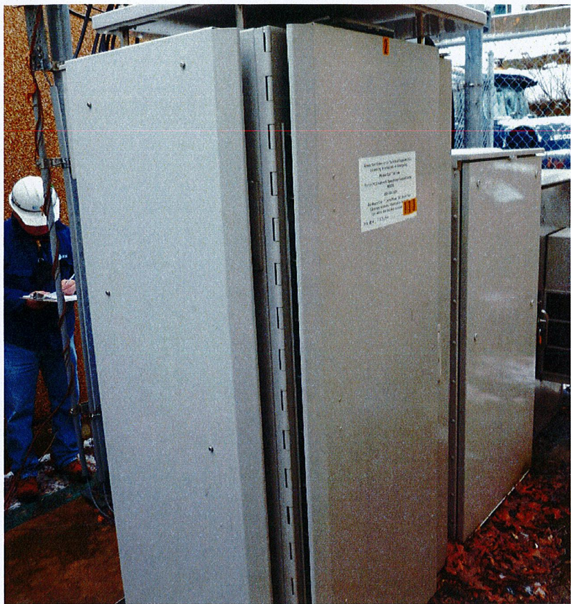
3 EXISTING EQUIPMENT AREA
