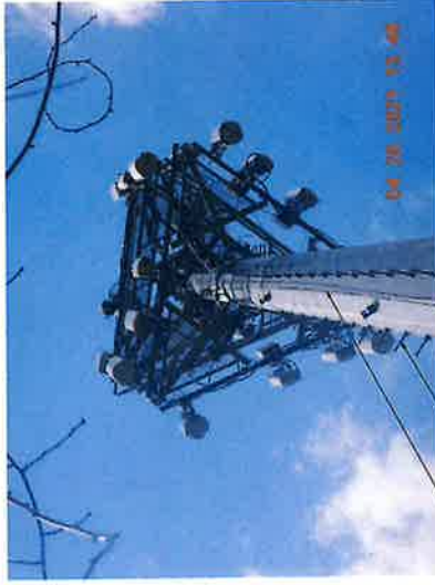
CLIMBING FACILITY PHOTO Existing Safety Climb Existing Climbing Facility
