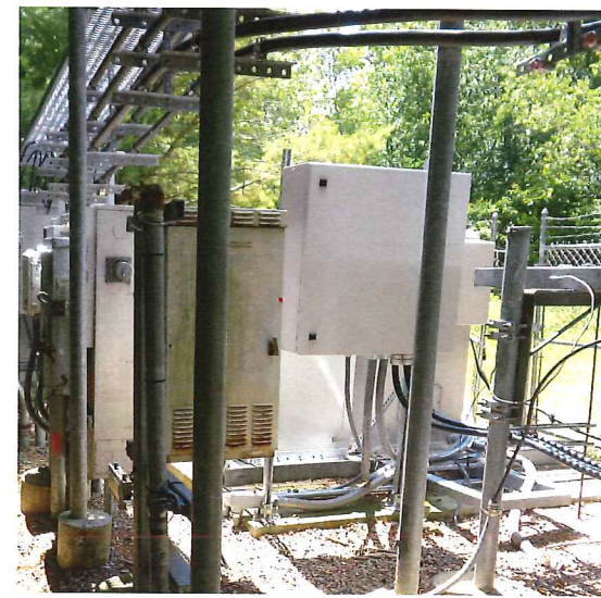
4 EXIST FIBER DISTRIBUTION BOX SCALE: NTS
