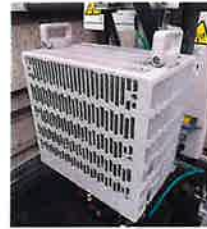
SAMSUNG RF4440d-13A B5/B13 RADIO DIMENSIONS: 15.0"H x 15.0"W x 9.0"D WEIGHT: 70.3 lbs QUANTITY: 1 PER SECTOR, TOTAL OF 3 SECTORS: ALPHA, BETA, GAMMA
